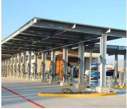
The WhiteWater Car Wash portfolio proves that even utilitarian buildings can be well designed and look great. The building design is both contemporary and playful, utilizing a number of materials including exposed steel, split face CMU, and stained wood planks. The canopy structure is designed with single column supports and large cantilevers to maximize the ease of traffic circulation in and around the site.
